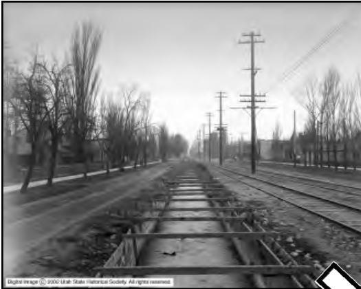
1900s: North Temple as a residential street, with City Creek running down the middle.
