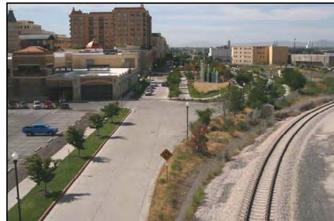
Looking south at the Gateway and 500 East from the viaduct.
